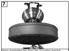
Hang assembled fan from the mounting bracket installed to ceiling in previous step. Make sure the fan is hanging straight. Rotate fan until the tab on the Mounting bracket engages the slot on the Downrod Ball. This must be done to prevent the fan body from rotating when the blades are in motion.
